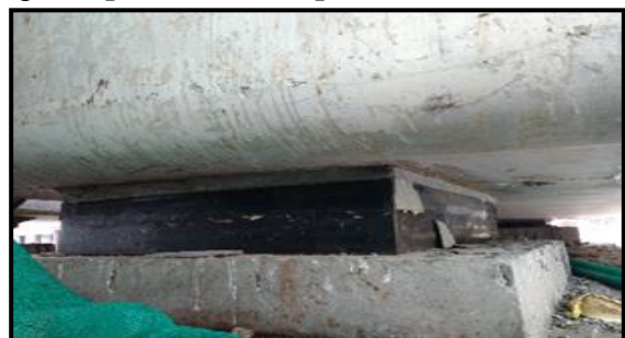
Fig. 3 –Grout placed above the bearing
