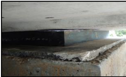
Fig. 5 – Grinding the surface and thin layer of grout below bearing
