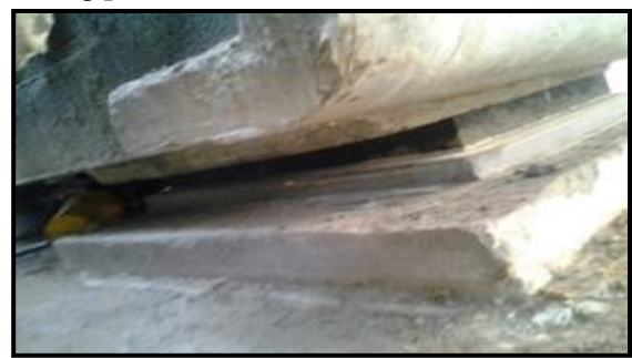
Fig. 1 -Placing the grout above the bearing (Fig.2)
