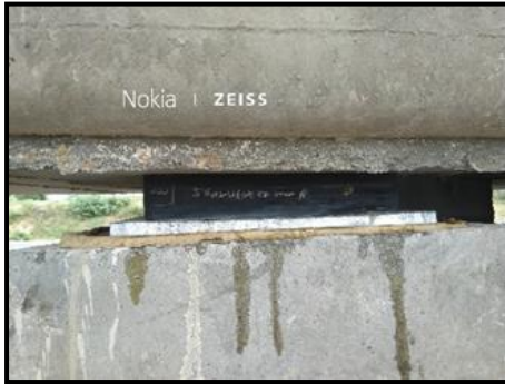
Fig. 4 – Steel Plate below bearing
