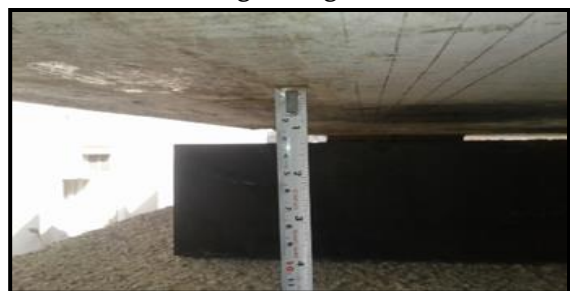
Fig. 2 –Space created to pour the micro concrete
