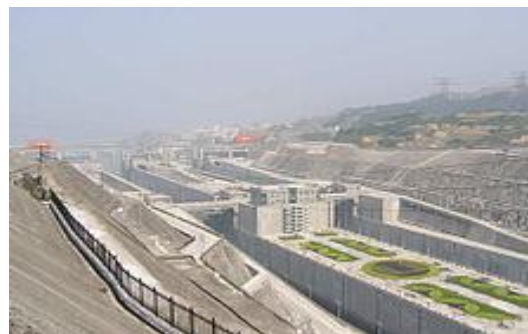
Fig-3: ship locks for river traffic to bypass the TGD
