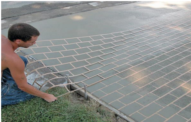
Fig-3: Removing of stencil layer
