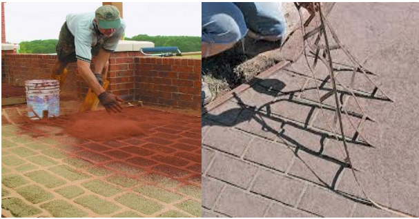
Fig-2: Laying of stencil concrete
