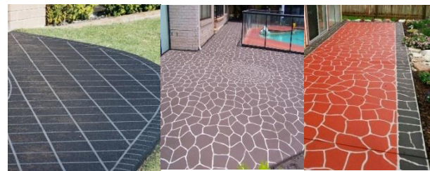
Fig-1: Stencil Decorative concrete
