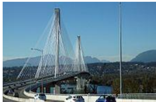
Fig-2: New Port Mann bridge
