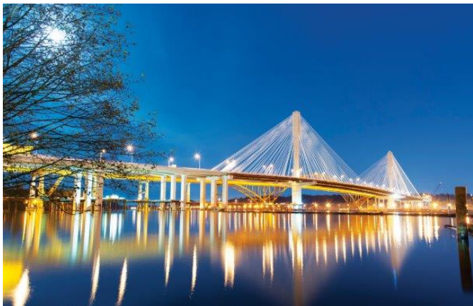
Fig-3: Port Mann bridge
