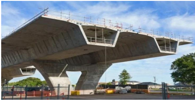
Fig 1 Precast Segmental Bridge
