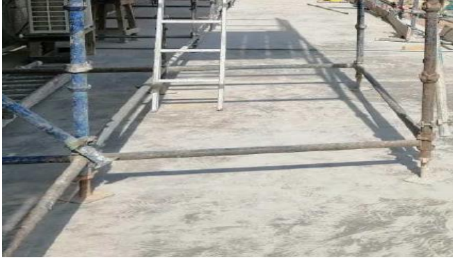
Loading platform slab
