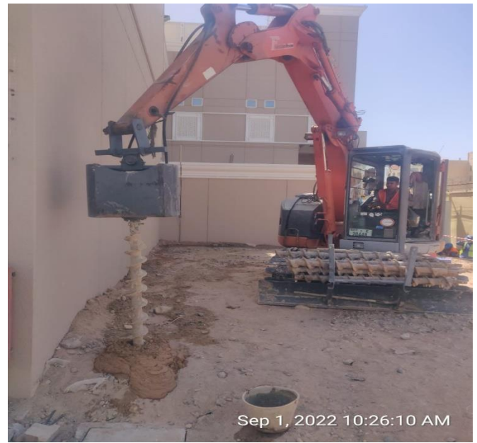
FIGURE 2. PRE-AUGURING TO CREATE VOIDS IN SOIL STRATA
