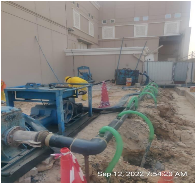
FIGURE 1. WELL POINT SYSTEM INSTALLED AROUND THE PERIPHERY
