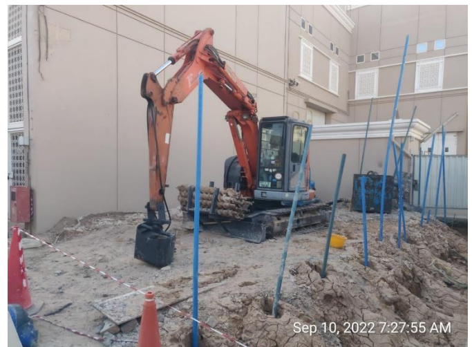
FIGURE 3. 50MM UPVC PIPE PLACED IN JETTING HOLES
