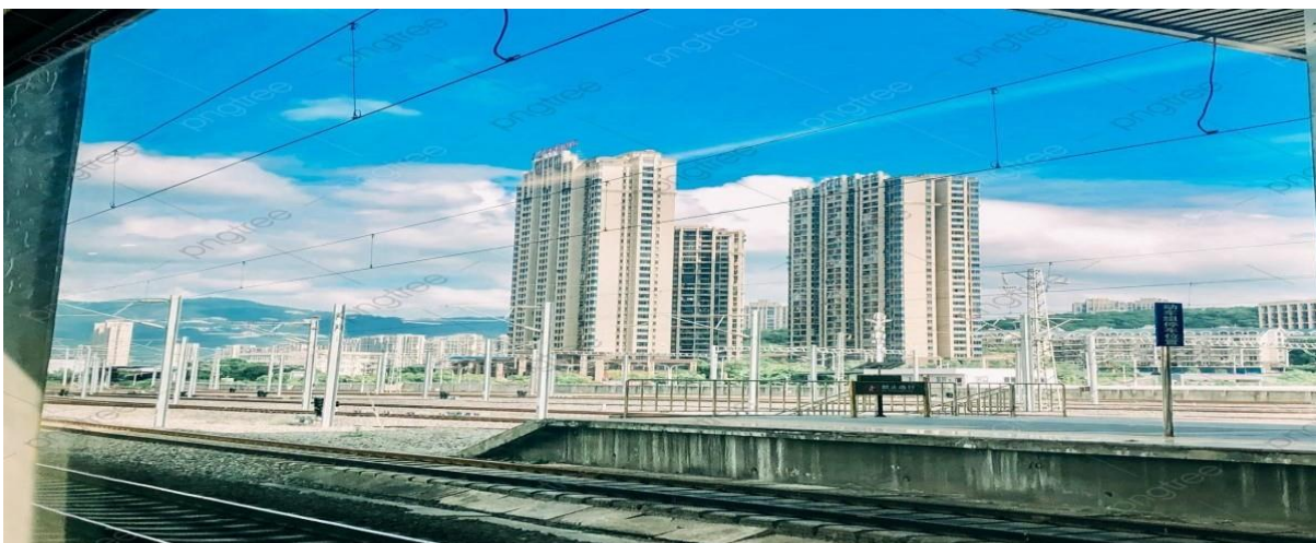
Fig 1 Structure nearby railway track
