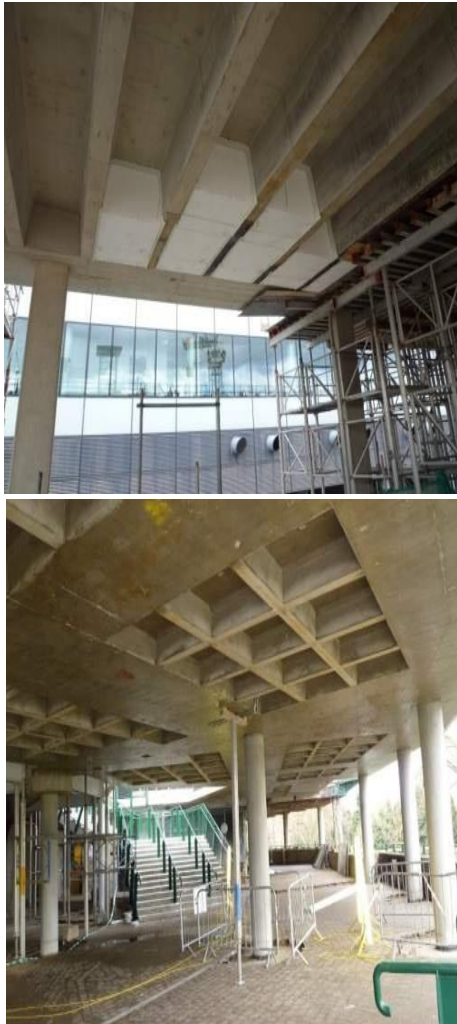
Fig 2 One way and Two way Ribbed Slab
