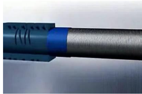
Fig-6: coating of main cable
