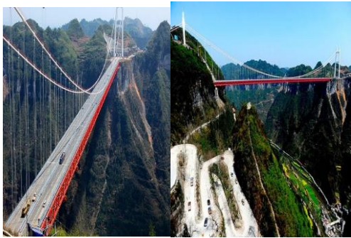
Fig-1: Aizhai Suspension Bridge
