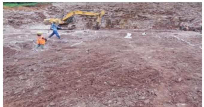
Fig: 2 Levelling of the site
