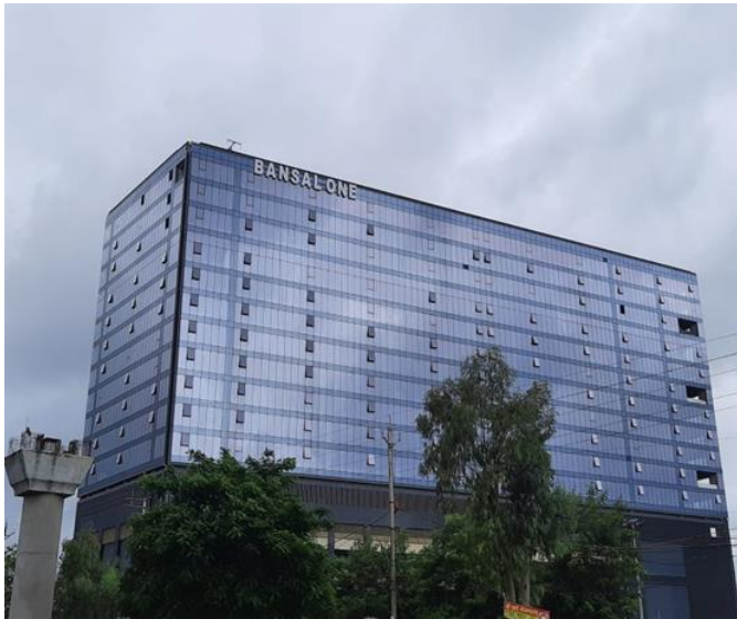
Fig 5 Actual Building final stage from the site Collection - Information Data General project information is given in Table 1. Table 1 : Project Information
