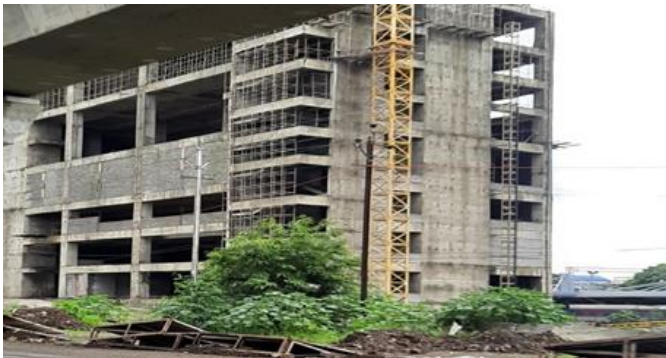
Fig 3.3 building after partial completion
