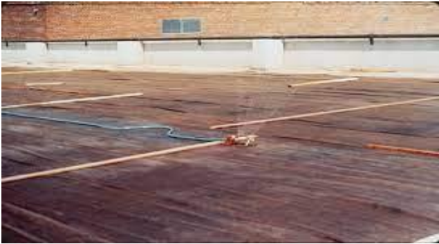
Figure 15. Curing using gunny bags
