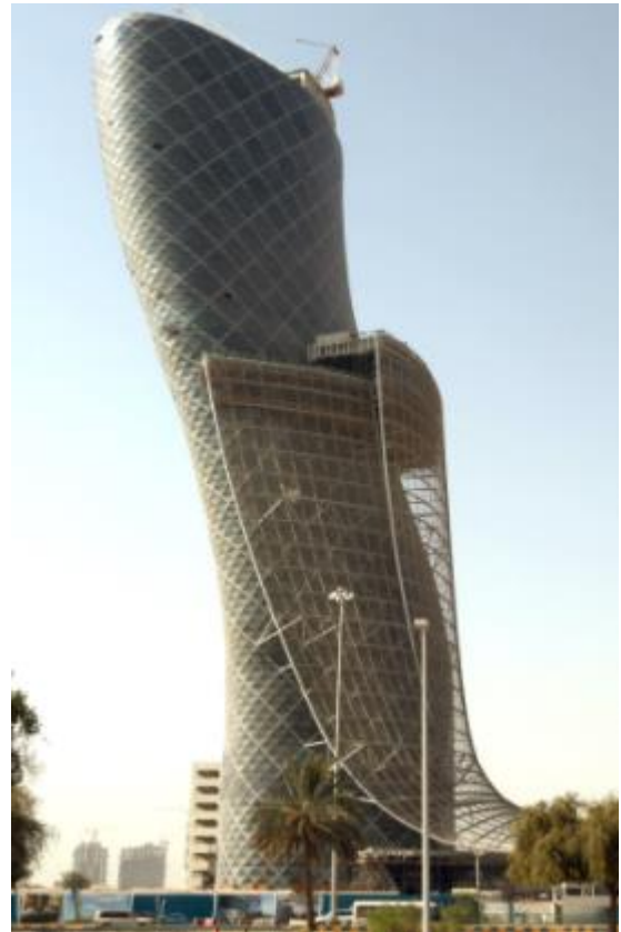
Fig 2 Tilted Tall Structure
