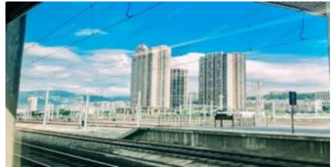
Fig 1. Structure nearby railway track Methods of analysis of structure
