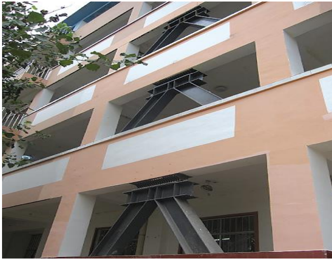
Fig 8 Metallic Yielding Damper Installed in Multistorey Building
