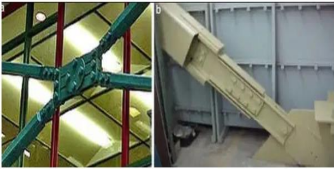
Fig 4 Friction Damper
