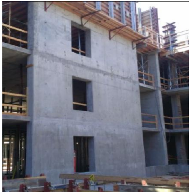
Figure 1: Example of RCC Shear Wall
