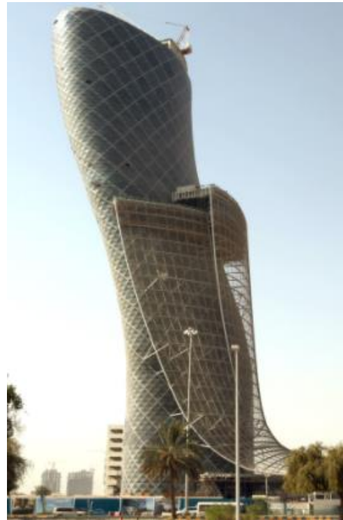
Fig 2 Tilted Tall Structure
