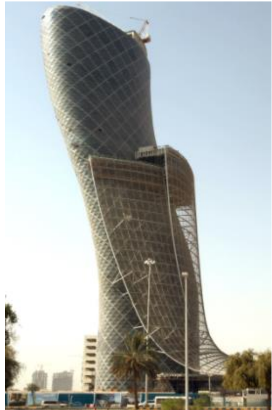
Fig 2. Tilted Tall Structure
