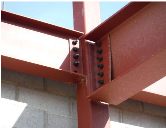
Fig 1 Bolted Framed Connections
