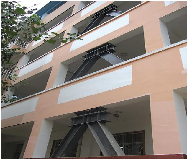
Fig 8 Metallic Yielding Damper Installed in Multistory Building
