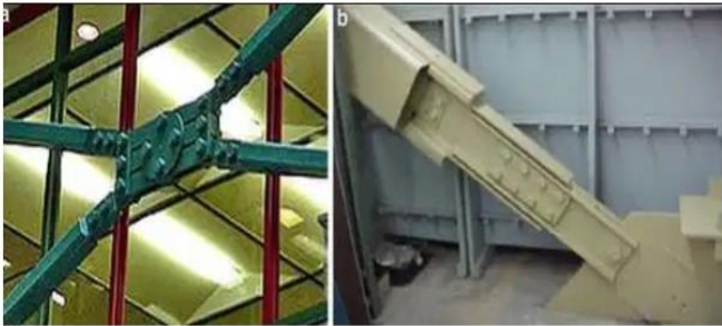
Fig 4 Friction Damper
