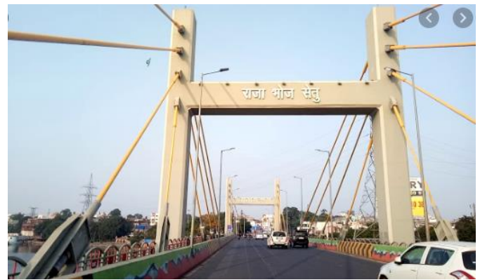
Fig 3 : Cable stayed bridge
