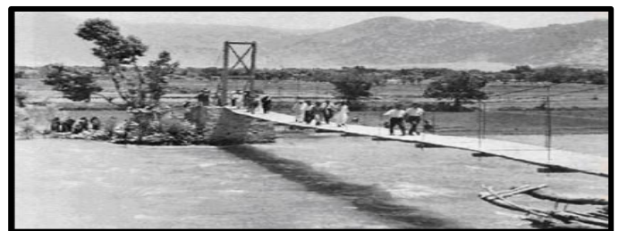
Fig 1 : Old Bridge structure
