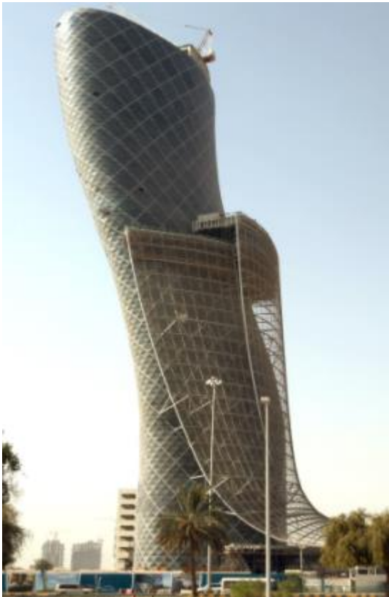
Fig 2 Tilted Tall Structure
