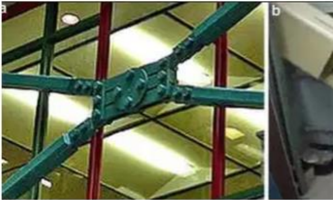
Fig 4 Friction Damper
