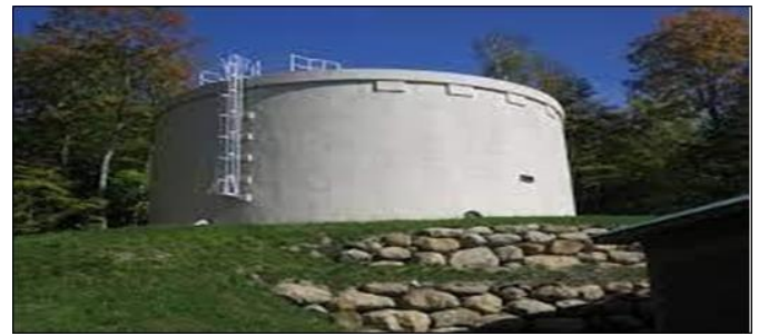
Fig 1 RCC water tank on earth surface Underground Water Tank
