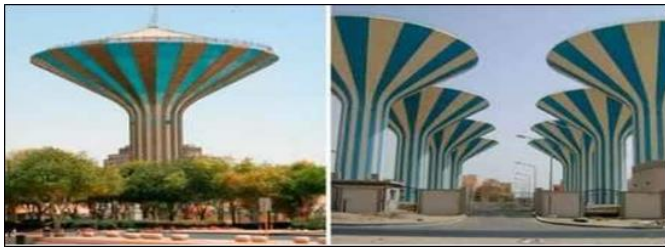
Fig 3 Elevated RCC water Tank
