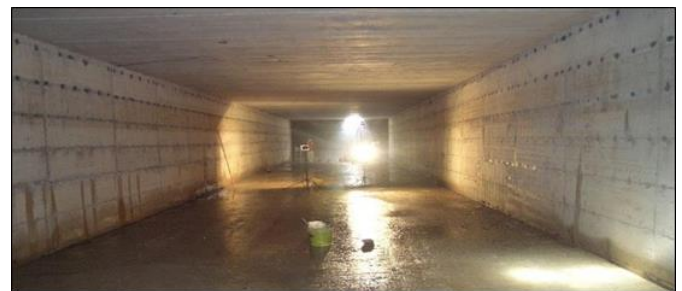
Fig 2 Underground Water Tank
