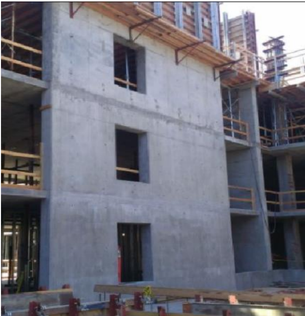
Figure 1 : Example of RCC Shear Wall
