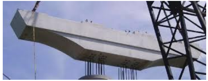
Fig 1 Precast Segment Structure
