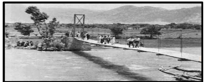
Fig 1 : Old Bridge structure
