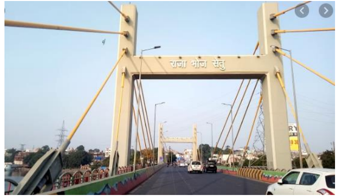
Fig 3 : Cable stayed bridge
