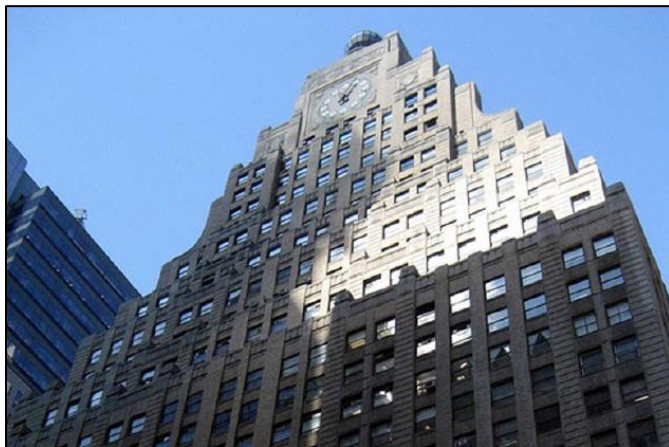
Fig 1 : The Paramount Building at New York, United States
