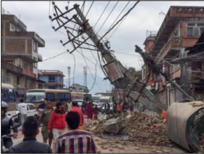
Fig 1: Seismic Failure in India (Assam)
