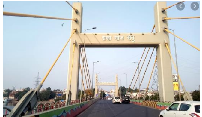
Fig 3: Cable stayed bridge
