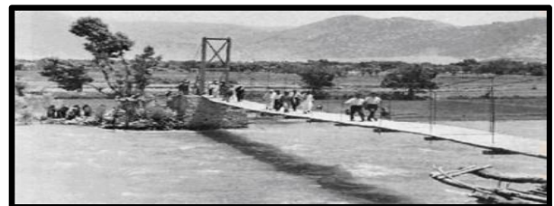
Fig 1: Old Bridge structure
