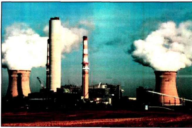
Figure 1. Self-supporting Steel Chimney
