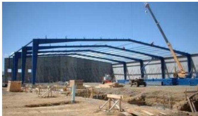
Fig 1. Steel Frame structure
