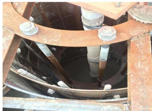
**Fig-5: Drilled shaft anchors**
