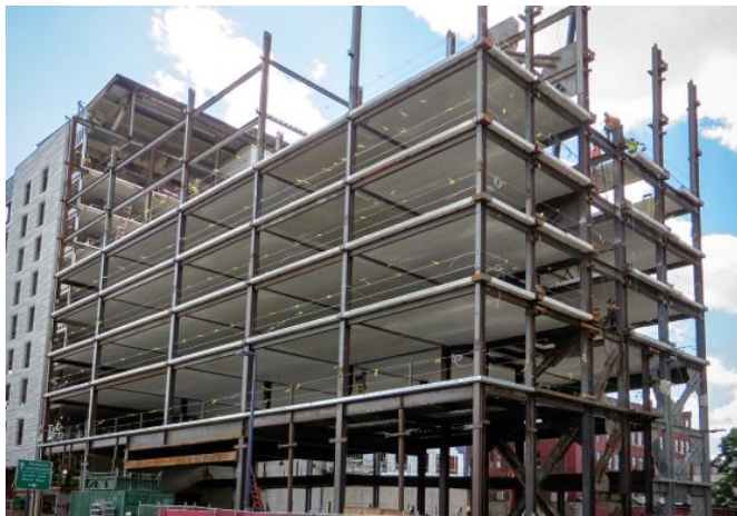
Fig 1 : Structure with slab
