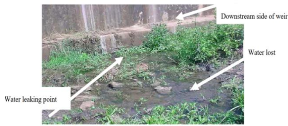
Figure 4. Leakage on River Diversion structure
