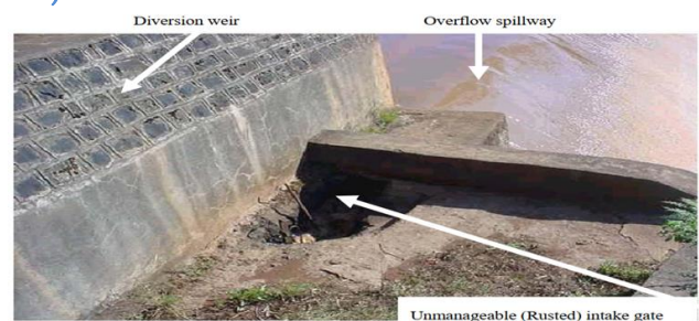
Figure 1. An intake gate of diversion head work The deposition of soil and debris can affect the functioning of a structure. For instance, a stilling basin collects soil deposits the available water mass diminishes and energy dissipation will be less effective. Similarly, in the case of soil deposits in a flow division
