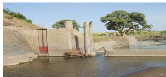
Figure 3. Part of River Diversion head work
