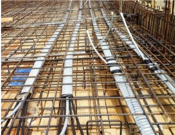
Fig 2 : Post Tensioning Slab
