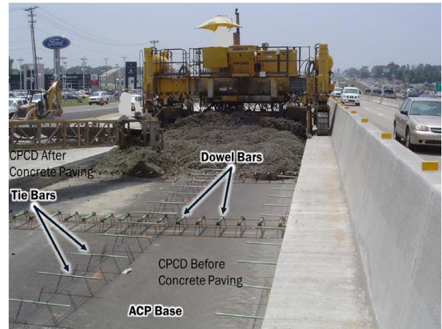
Figure-1: Typical section of rigid pavement
